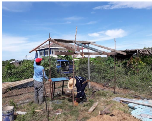
SSVTC personnel during the construction of Pig pen
