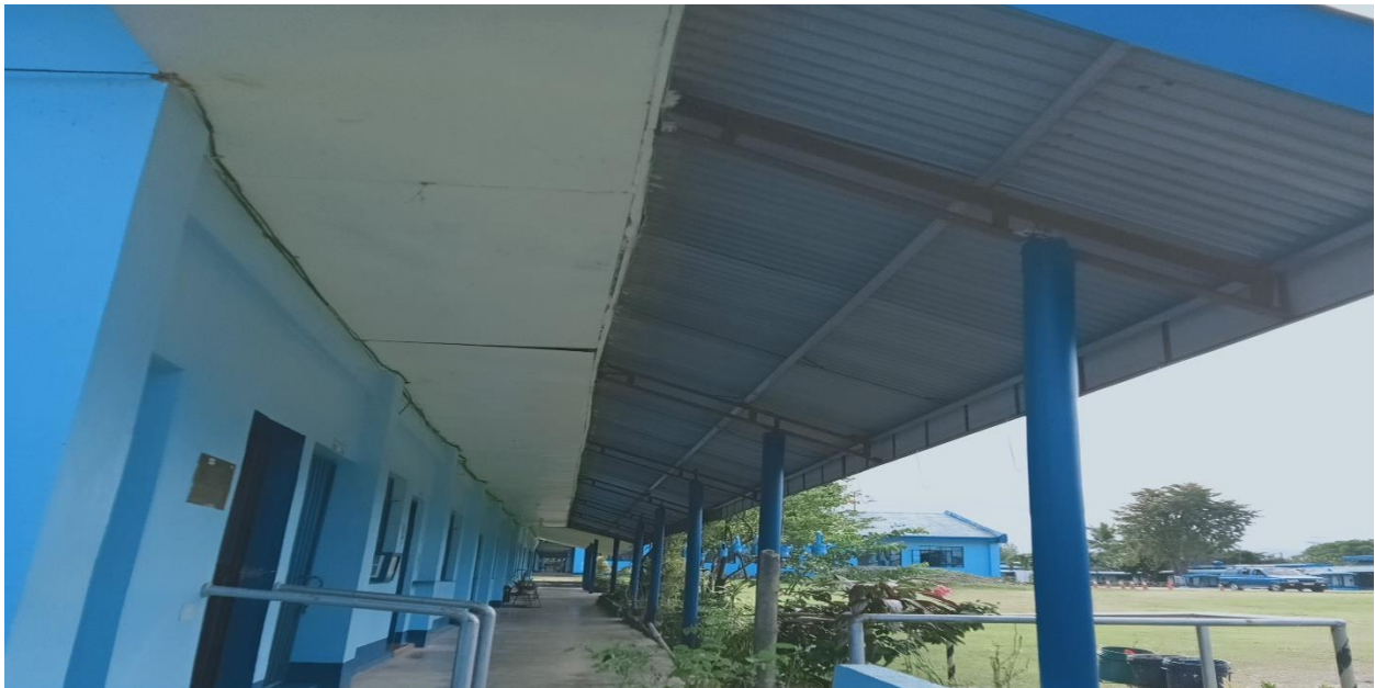
Housekeeping building with extended roof for pathway cover.
